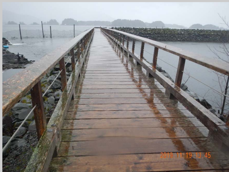
Example of a yellow cedar elevated boardwalk constructed in Phase I.
