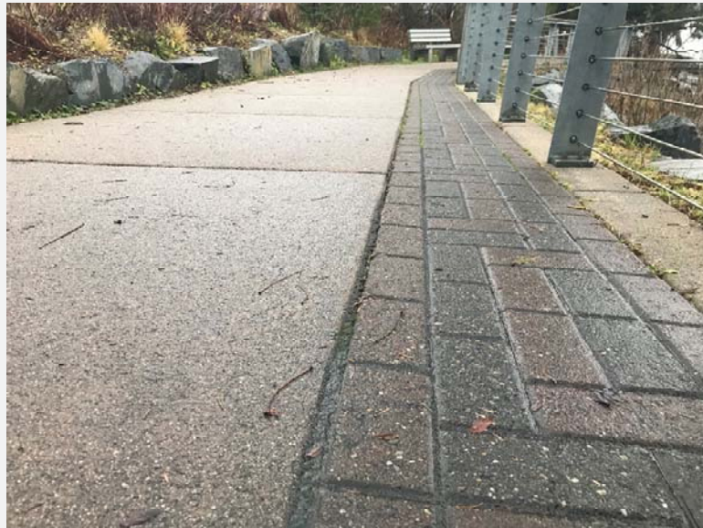
Example of the “red brick road” constructed in Phase I.
